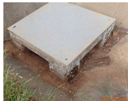
Main drain inlet at Hager and Coolidge
